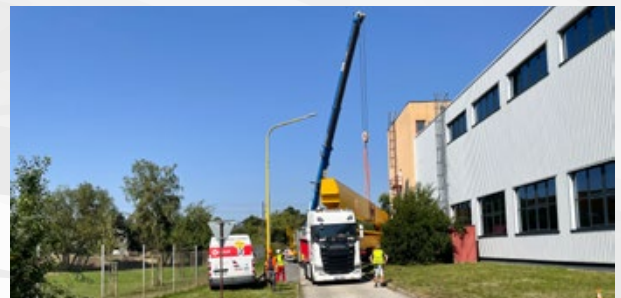
The new crane is delivered by heavy-duty transport.
