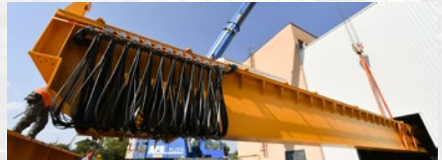
Moving into the hall.
